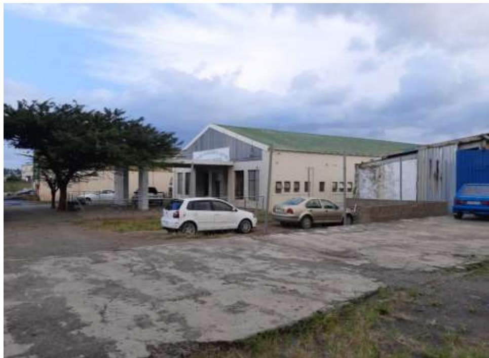
Diagram 8: External view of the original Disaster Management Centre, that is now used as an Auditorium venue and the informal parking area.
