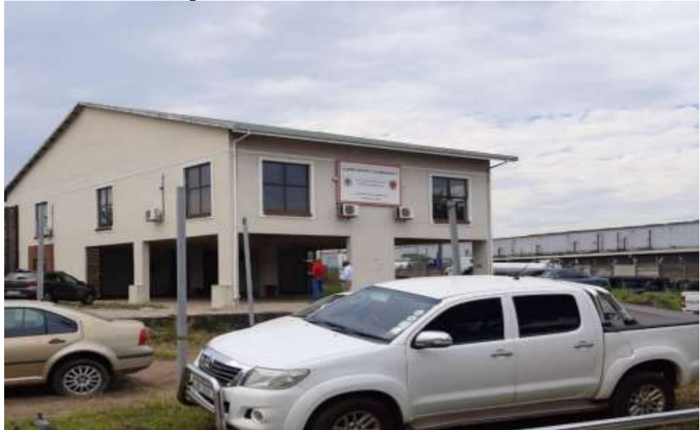
Diagram 5: External view of the DMC from the carpark and the unused open ground floor space within the DMC, which lends itself to office space conversion. This is also the only access and exit point to the building.
