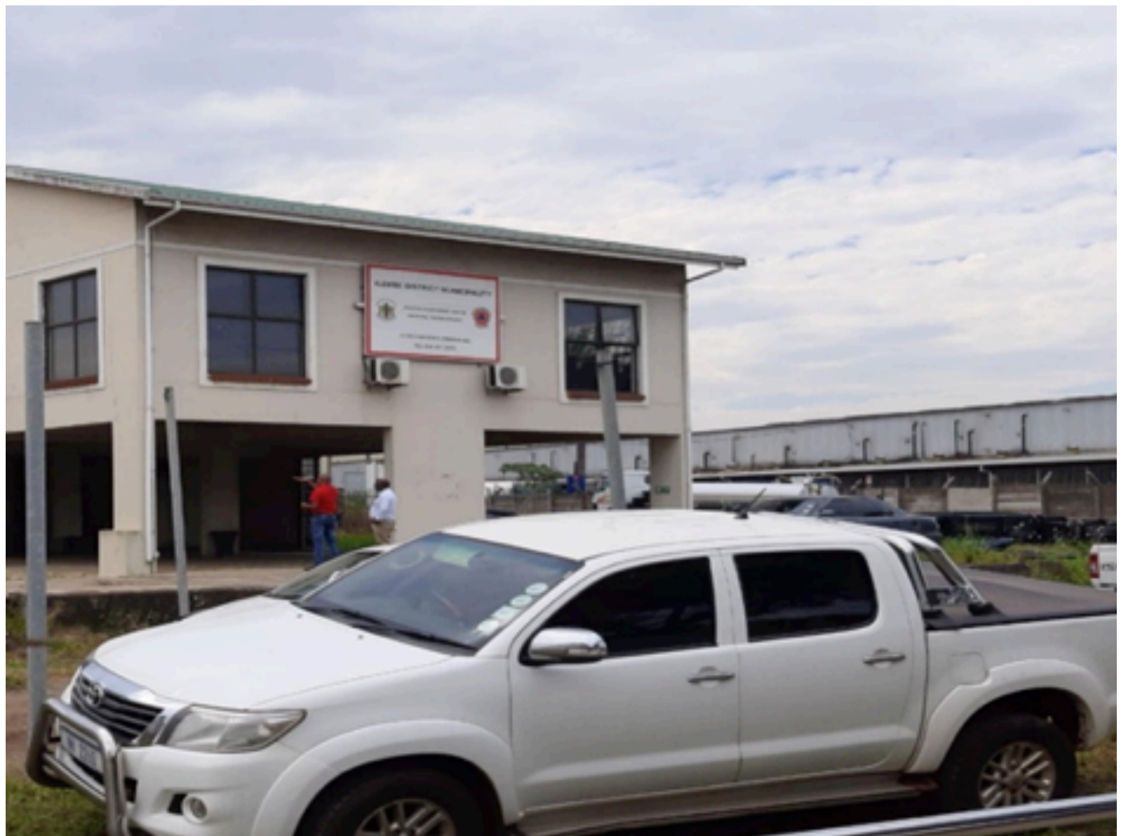
External view of the DMC from the carpark and the unused open ground floor space which lends itself to extended office space
