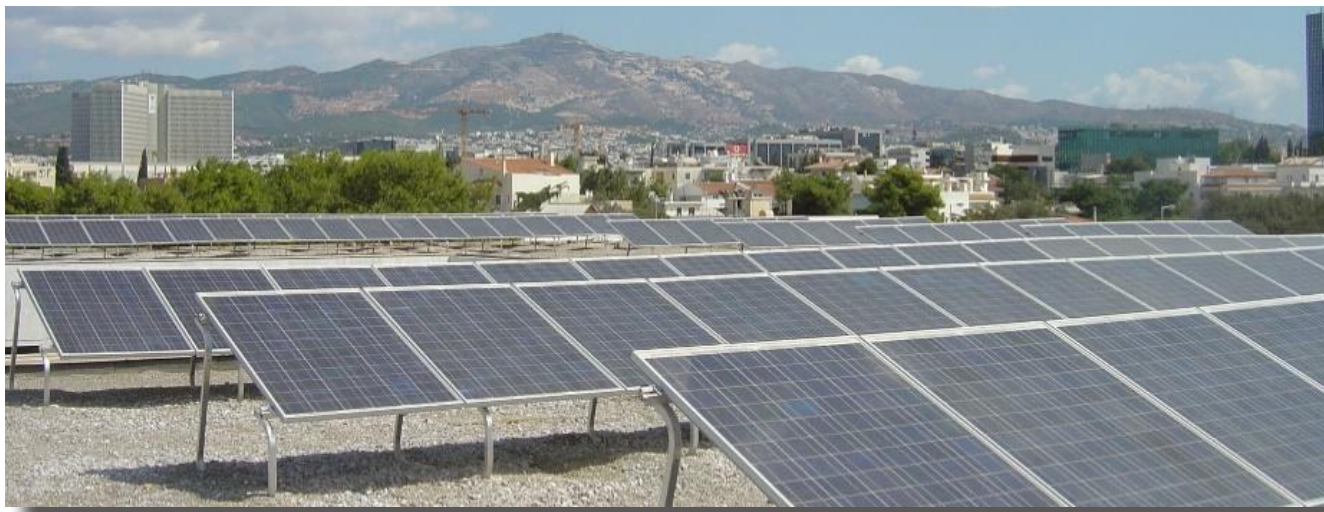
Rooftop solar installation
