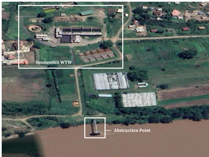
Figure 5: Site overview (Source: Google Earth)
