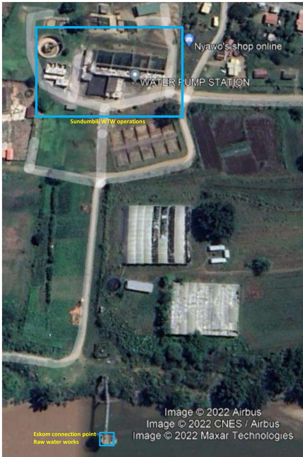
Figure 25: Raw water work connection point
