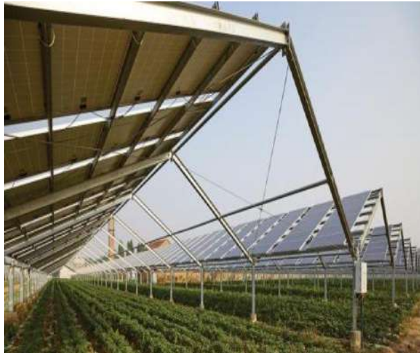
Figure 38: Agri-PV mounting structure [8]
