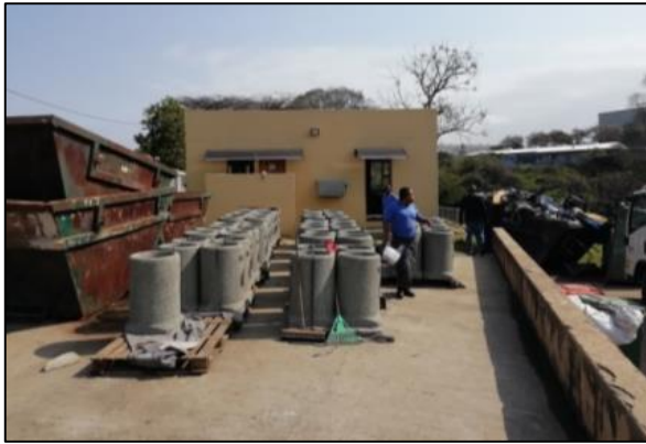
A: Storage of street bins and skips at the Transfer Station
