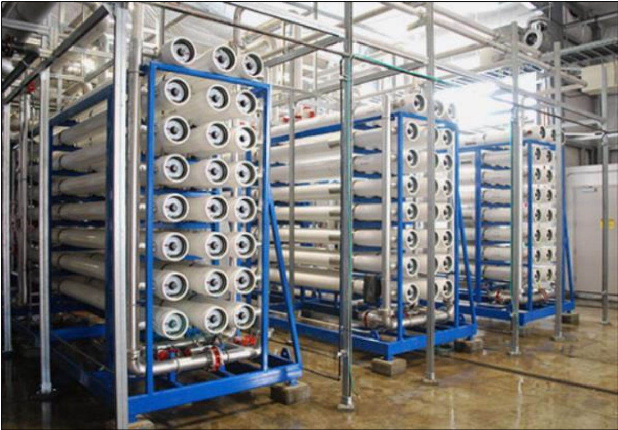
Figure 15: Skid mounted membrane pressure vessel installation
